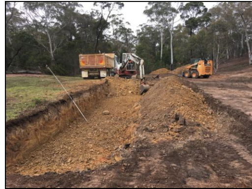
Digging digging digging
